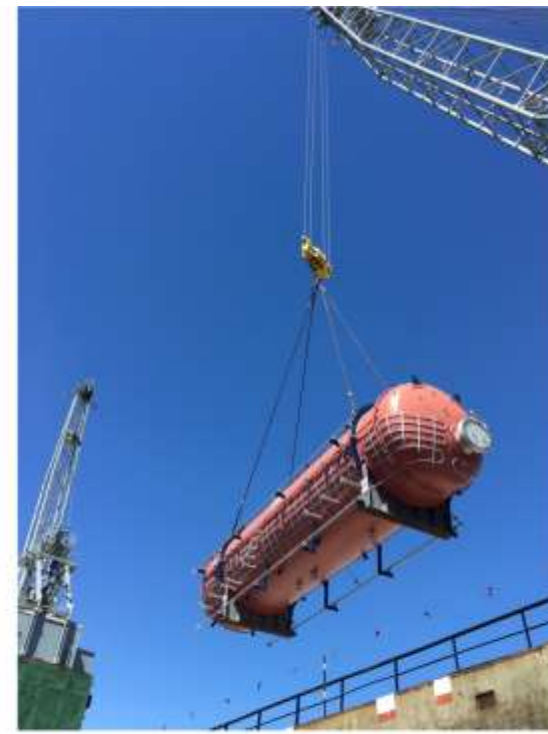
#33 Dessalter Vessels & spare parts Thessaloniki to Russia 14.50 x 3.60 x 4.20 mtrs / 36T Scope: ex works till FOB Thessaloniki
