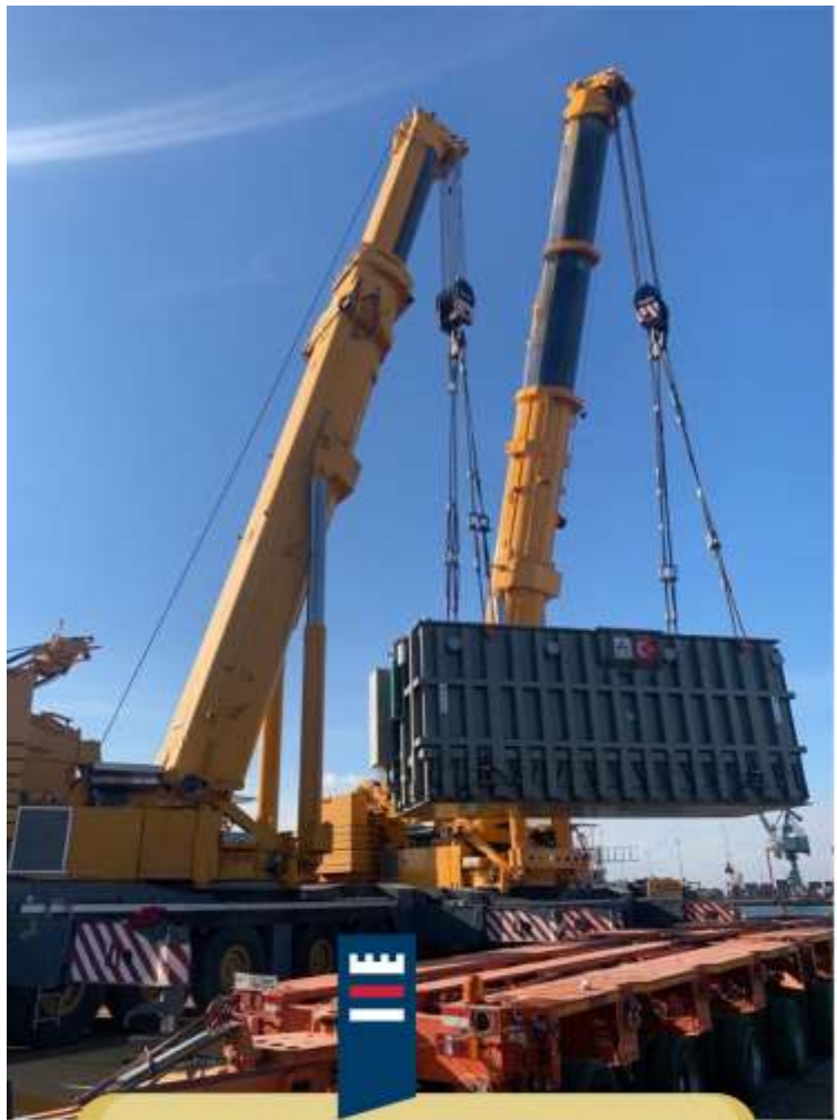
E #24 Power Transformer 280 MVA/400 1 x unit 10095x4120x4315mm / 240T Thessaloniki port Scope: FOB till FOT & transit customs formalities to NMK
