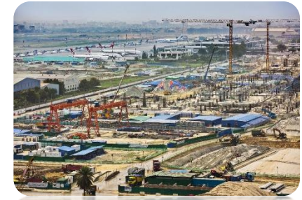
Dhaka Airport Expansion Project
