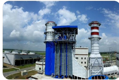
Rupsha 800-Megawatt Combined Cycle Power Plant Project
