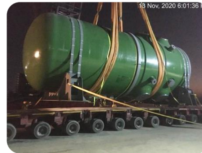
Handling Reactor Pressure Vessel
